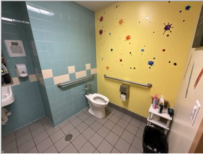
TOILET STALL OVERVIEW
