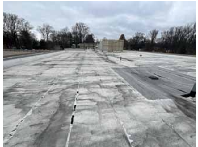
10 - SECONDARY ROOF OVERVIEW
