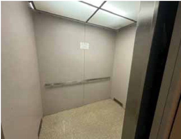
21 - ELEVATOR CAB FINISHES
