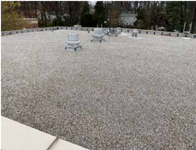
9 - PRIMARY ROOF OVERVIEW
