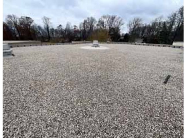
8 - PRIMARY ROOF OVERVIEW
